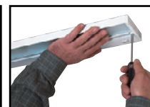
Step 3 Mount fixture to cabinet bottom using captive mounting screws.
