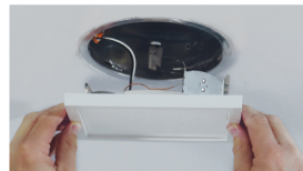
Friction clips for recessed housings
