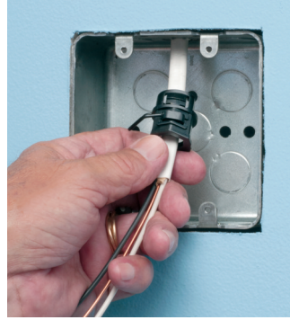
Push assembly into box...
