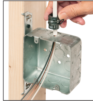
Push assembly through knockout...
