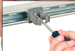
3 Tighten screw for secure installation on strut.
