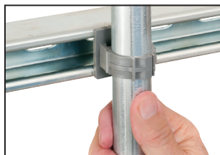
5 Secure installation of conduit to strut.
