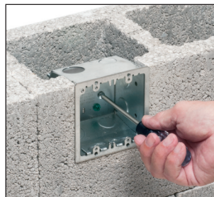
Tighten the screws on the spring clip to pull it securely against the block.
