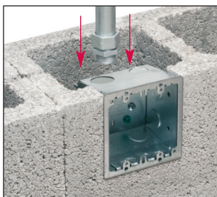
Install the EMT in the top of the box.
