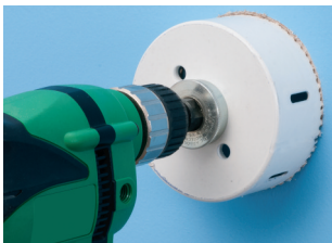
Determine sconce light location. Cut opening with 4" hole saw.
