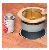
2 Wire receptacle per applicable local, state and national codes. After installation of finished flooring secure leveling ring assembly to installed concrete can using PVC cement.
