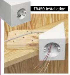
Cut a 2x8 approx. 18" long. Install FB450 on 2x8 allowing it to extend 8-10" past the box. Keep bottom of box level, short side of box touching angled rafter. Nail or screw assembly to rafter.
