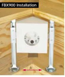
1 For proper fan/fixture installation, use supplied template to level and position brackets between rafters. Remove captive screws on sides of brackets and use to attach FBX900 assembly to rafters.
