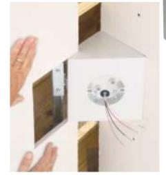
3 Cut and position drywall to fit around the box. (Note captive screws in box.) Install fan or fixture per manufacturer's instructions using captive installation screws.
