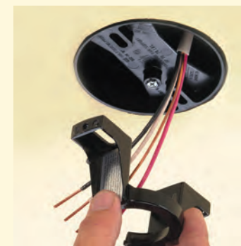
4 The fan/fixture bracket installs directly onto the joist through the oval slots in the box.
