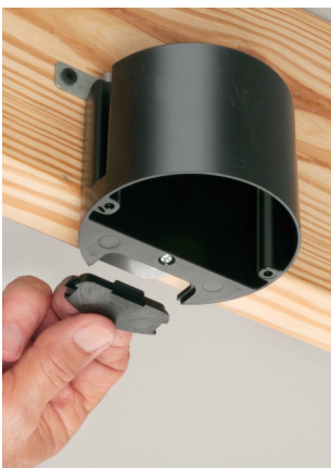
Photo A (cutaway) shows box set back in double drywall ceiling
