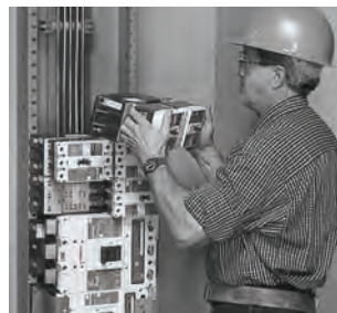
Panelboard Installation
