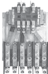
Socket and Test Block Assembly
