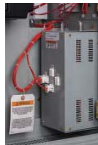
Multi-Tap Control Power Transformer
