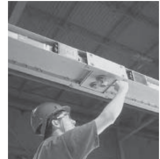
Typical Busway Installation (Torque Indicating Bolt)
