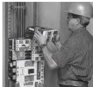
Panelboard Installation
