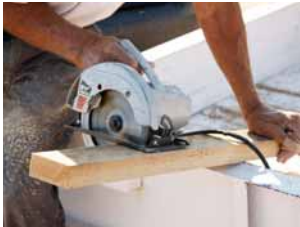
Construction Site Application
