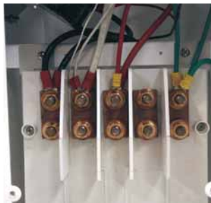
Copper Busbar with Ratings from 250 to 500 A
