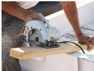
Construction Site Application
