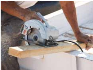
Construction Site Application
