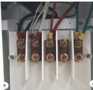
Copper Busbar with Ratings from 250 to 500 A
