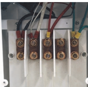
Copper Busbar with Ratings from 250 to 500 A
