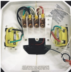
Copper Busbar with Ratings up to 140 A
