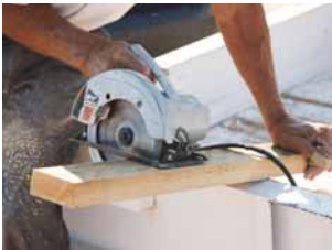
Construction Site Application
