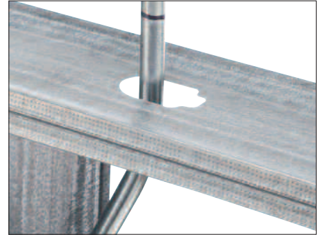
2 EMT marked and ready to cut.
