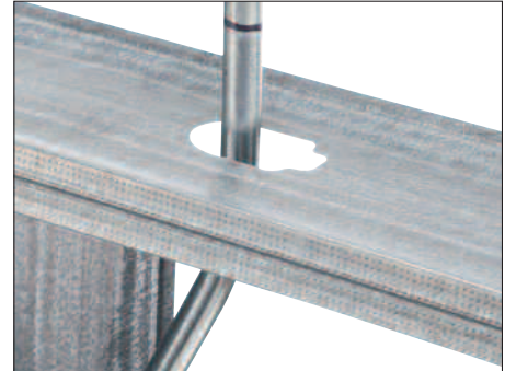
2 EMT marked and ready to cut.
