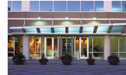
outdoor facility lighting
