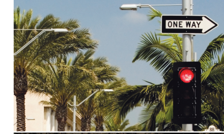
traffic signal controls
