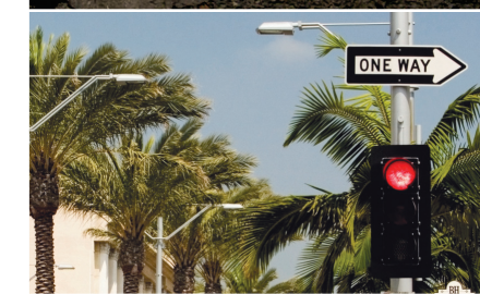
traffic signal controls
