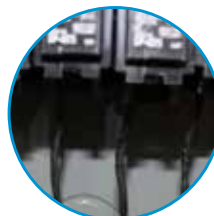
Improperly torqued circuit breaker lugs.
