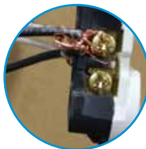
Improper stranded wire connection.
