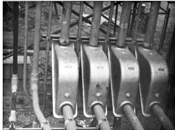
Conduit Systems Installations
